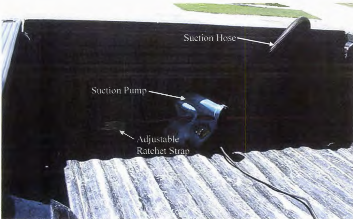
Figure 5.1.2. Suction pump secured by adjustable ratchet straps.
